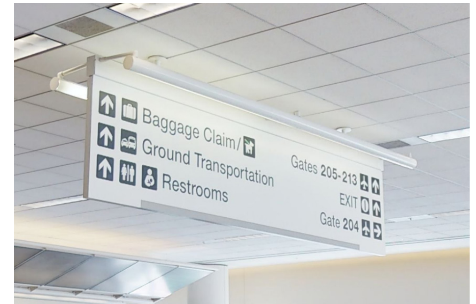
View of signage showing light fixture attachment
