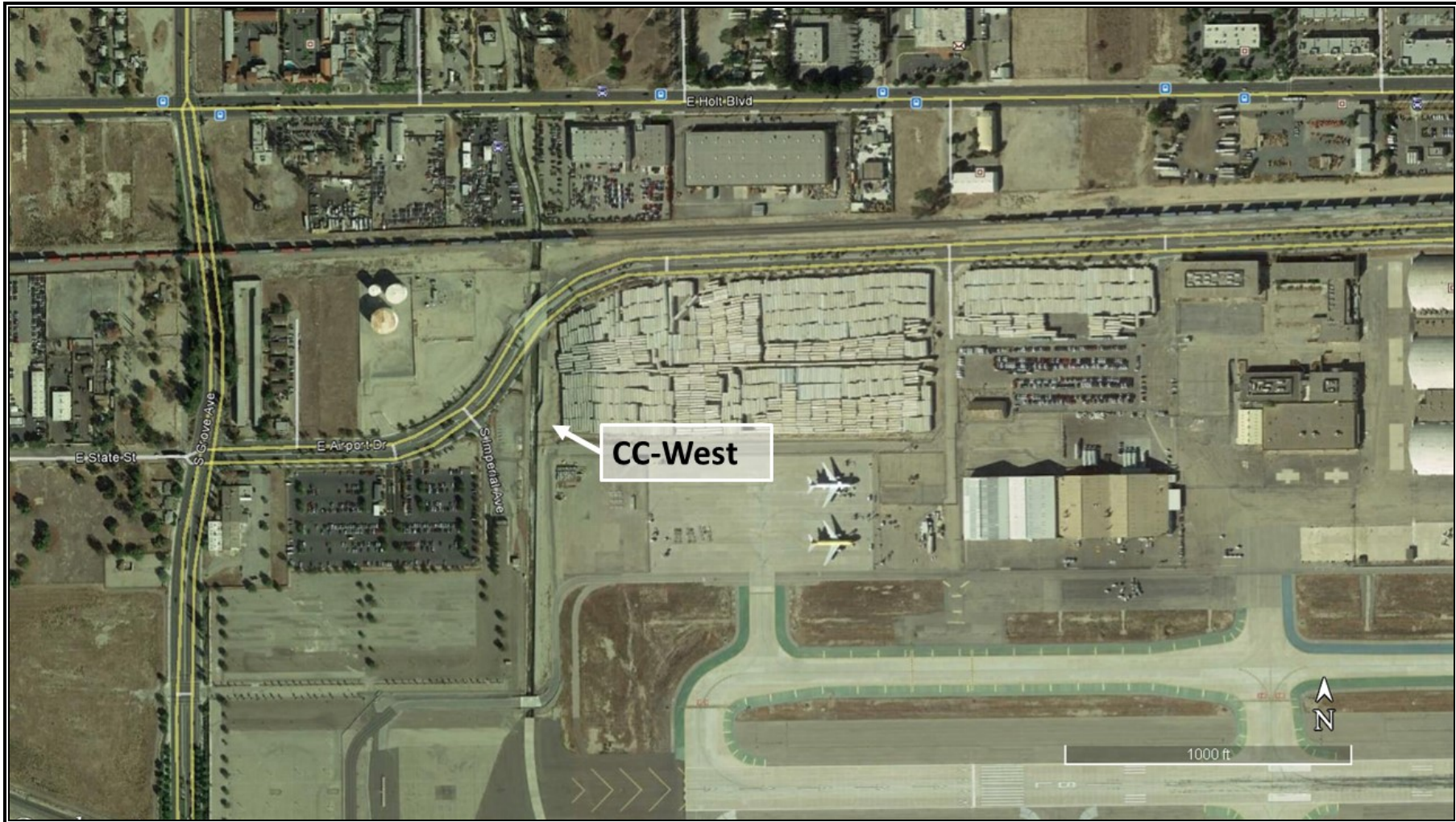
Figure 4. Cucamonga Channel West (CC-West) Monitoring Location.
