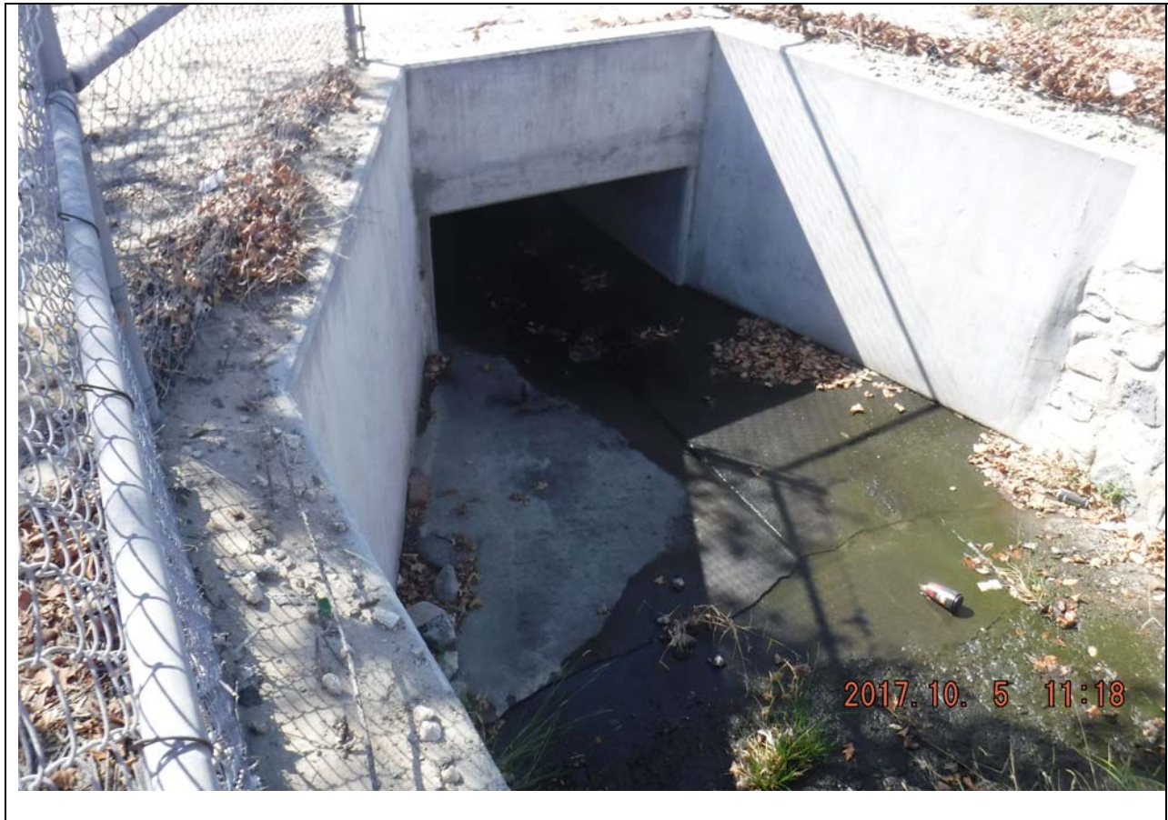
Figure 10. Photograph of Deer Creek Upper (DC-Upper) Monitoring Location.
