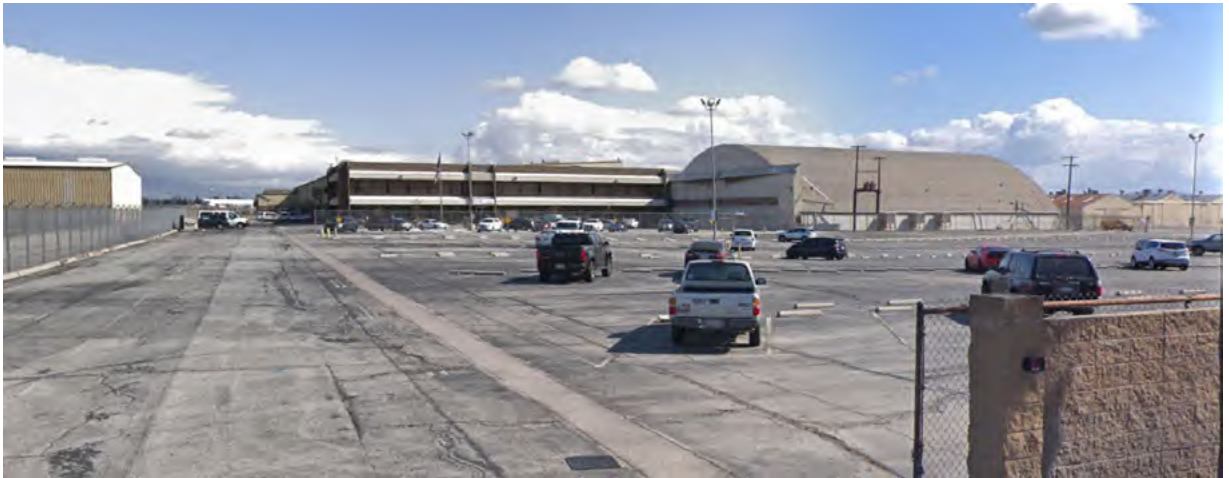
View of the OIAA Administration Offices at the southwest corner of the Project site on East Avion Street.
