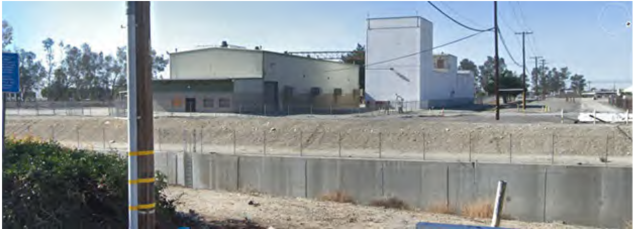
View of former GE buildings, south of the Project site at the Cucamonga Canyon Channel and future realigned East Avion Street.
