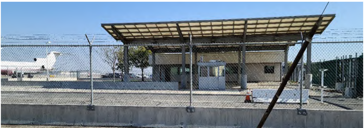
View of South SAAP facility.
