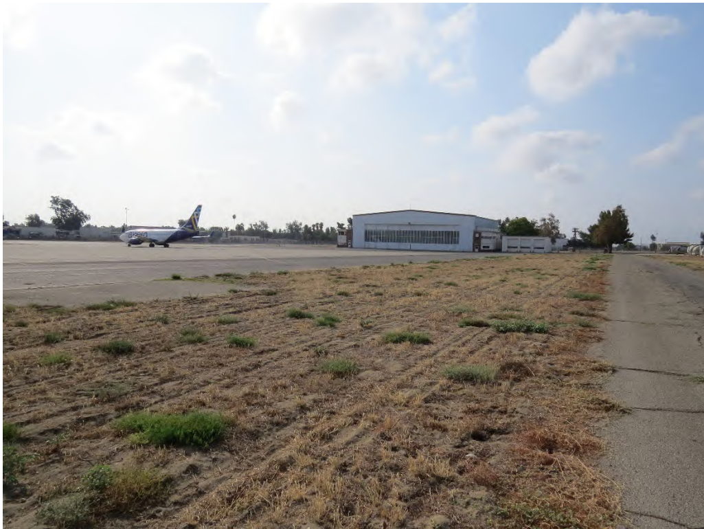
Photograph 12: Looking southeast at one of the disturbed areas on the eastern portion of the site.
