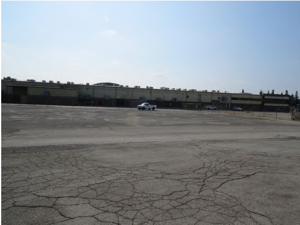
Photograph 5: From the northwest corner of the project site looking southeast.
